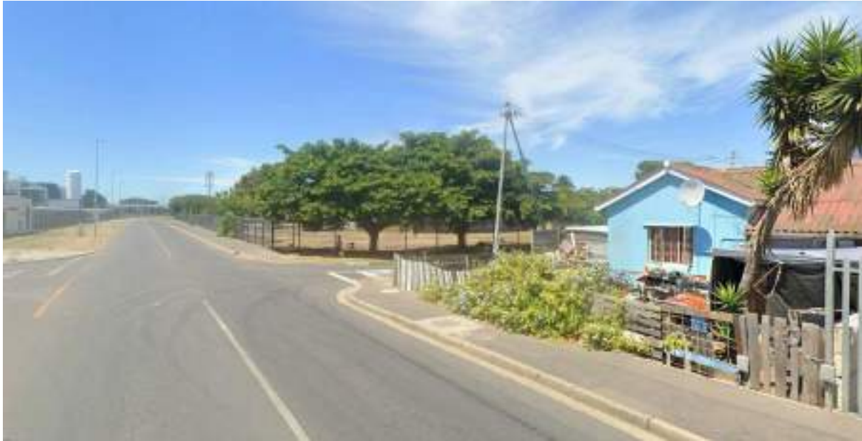
Figure 129: View B: Along Alexandra Road, looking South towards the train station.
