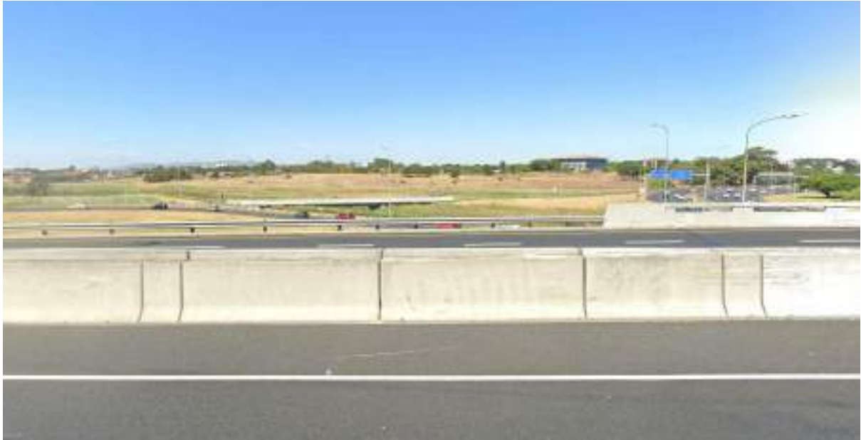
Figure 123: View E: Eastwards from the M5 bridge over the N2 across the Black River
