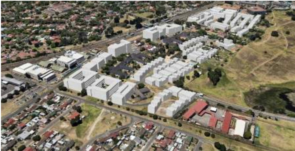
Figure 102: Alternative 4A: Aerial view looking towards the south. Source: SVA
