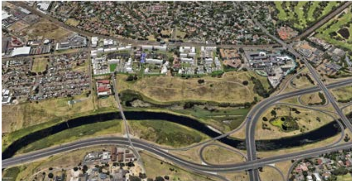
Google Earth Aerial View from the West
