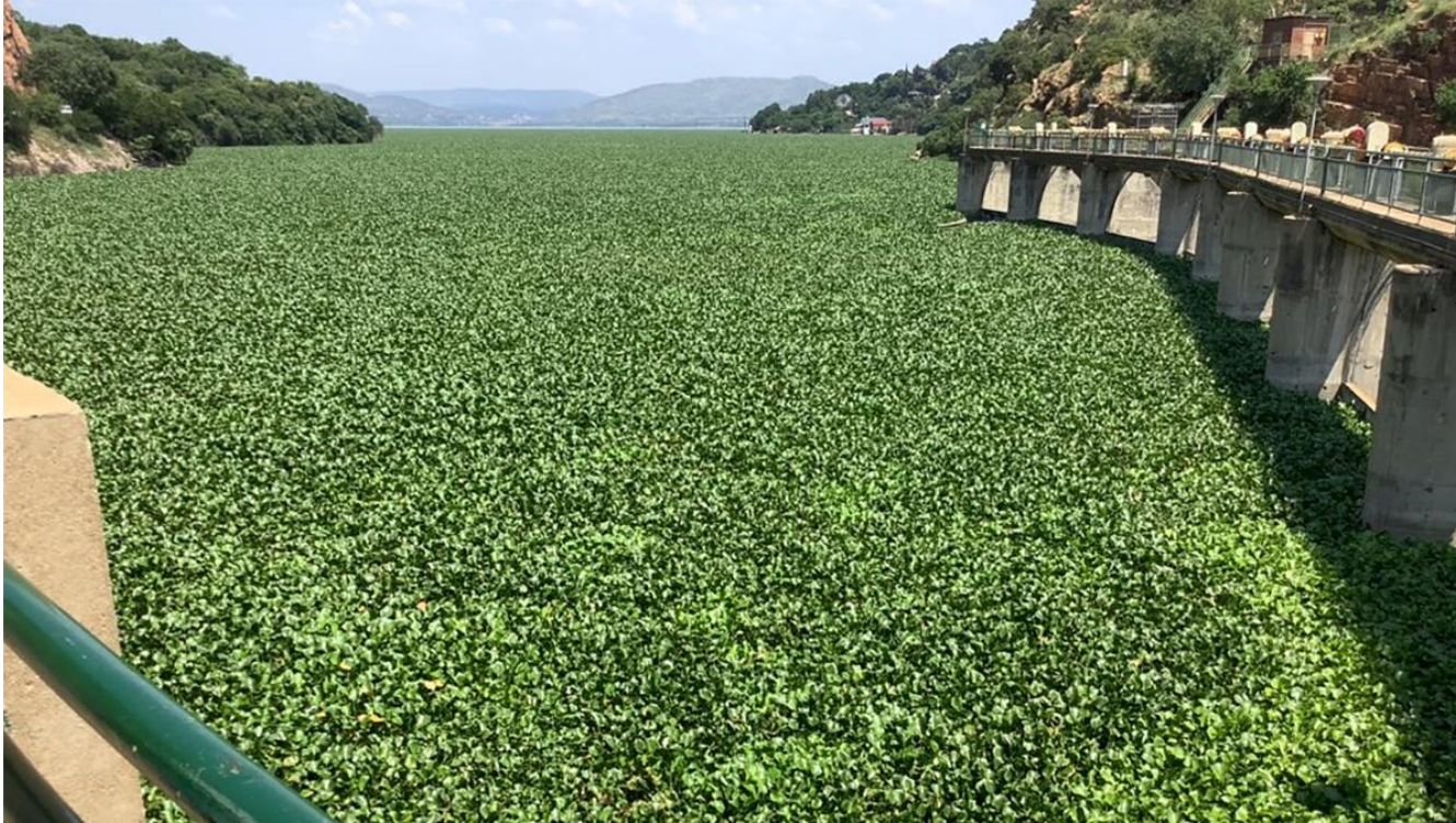
Hartbeespoort dam – hyacinth mat covers the surface due to pollution and poor water quality.
